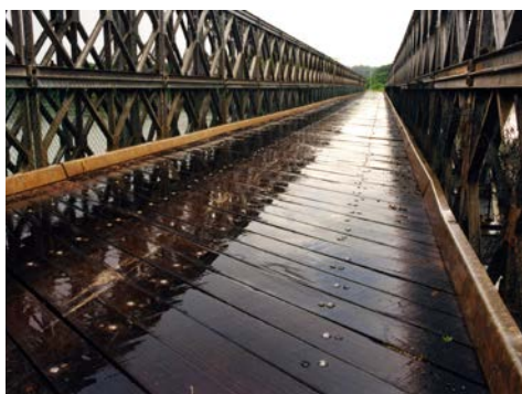
Decking on a bridge over Comté river (French Guiana).
