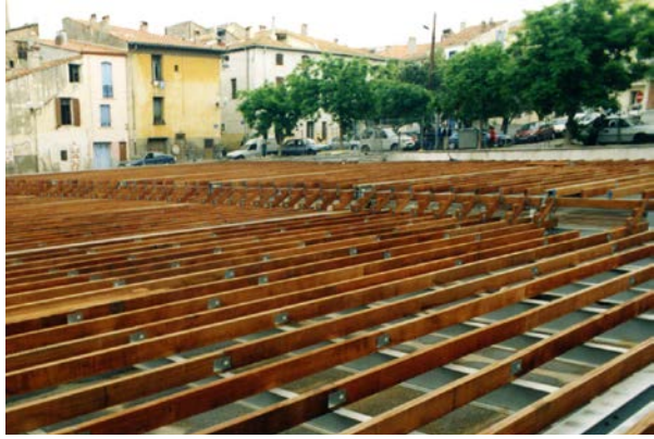
Sub-structure of the planking of the Forum Saint-Martin in Perpignan (France).
