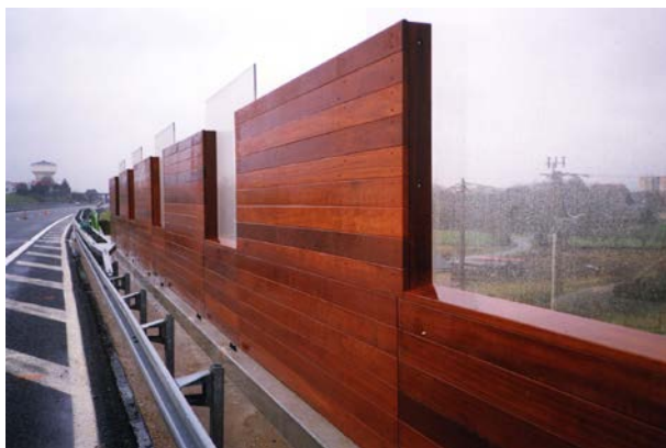
Sound protection screen, A10 motorway – Châtelleraut (France).
