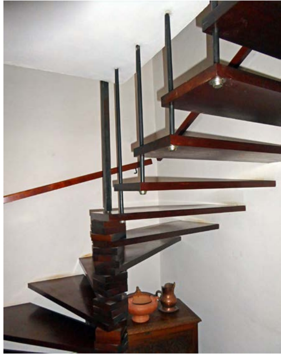
Semi-spiral, suspended staircase, Argelès-sur-Mer (France).
