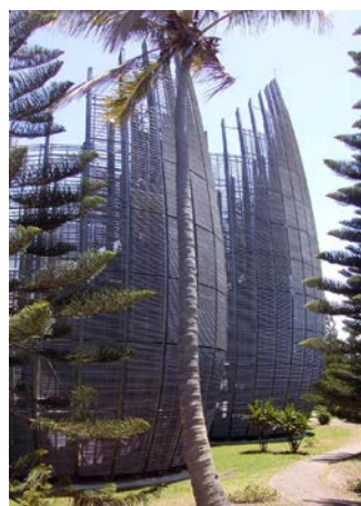
Glued laminated framework, Jean-Marie Tjibaou Cultural Centre – Nouméa (New Caledonia).
