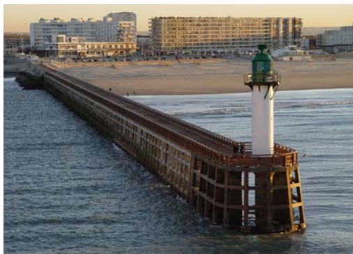
“Tillac” on the Calais pier – Design by Bois et loisirs (France).
