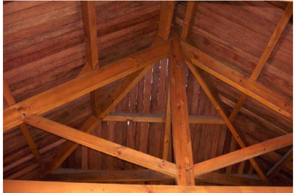
Coconut sheathing on ceiling frame ( Pinus caribaea ) (New Caledonia).
