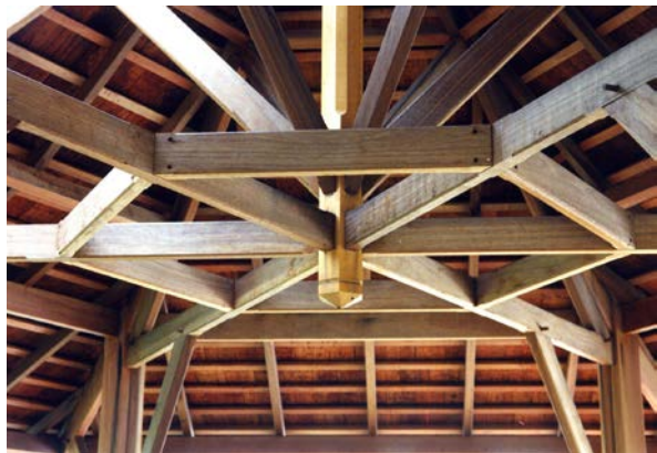
Traditional framework in Basralocus (shingles in Wallaba) – Kourou (French Guiana).
