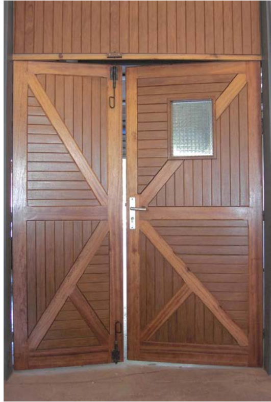
Utility door, CIRAD wood workshop, Montpellier (France).
