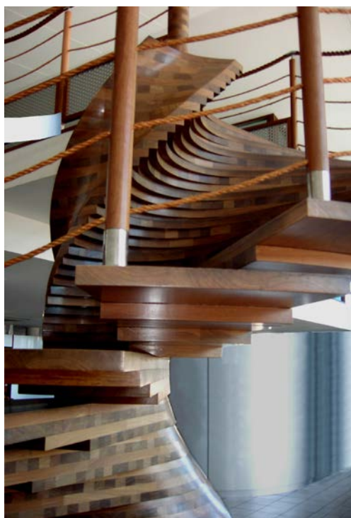
Interior staircase in glued laminated timber – by Les Bois du Pacifique, Nouméa (New Caledonia).
