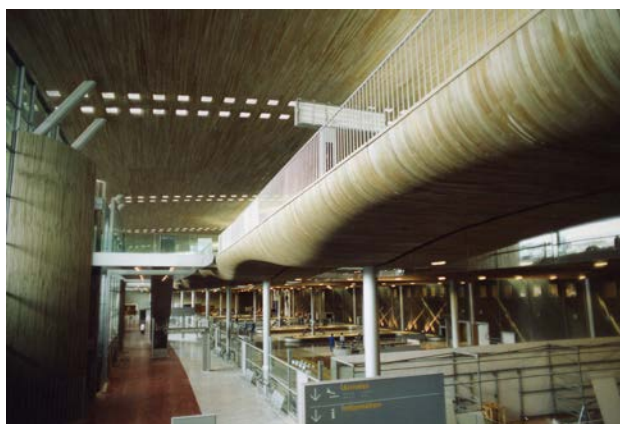
Ceiling of Paris-Charles-de-Gaulle airport in Roissy-en-France (France).
