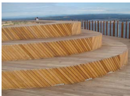
Decking on the belvedere of Mont Saint-Clair, Sète (France).
