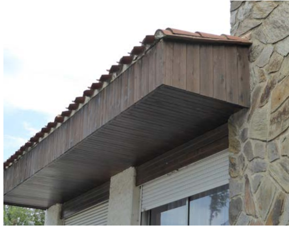
Cladding on roof overhang next to a stone-covered wall, Argelès-sur-Mer (France).
