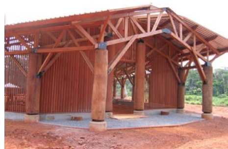
Posts in Tali (0.6 m in diameter, 8.5 m in length), door in Moabi, framework in Kosipo, vertical thin timber cladding in Mukulungu – J.Y. Riaux, Mindourou (Cameroon).
