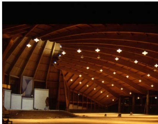
Glued laminated indoor structure at the Mary Queen of the Apostles Basilica in Yaoundé (Cameroon)
