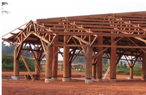
Triangular structure in Kosipo and posts in Tali – By J.Y. Riaux Mindourou (Cameroon).
