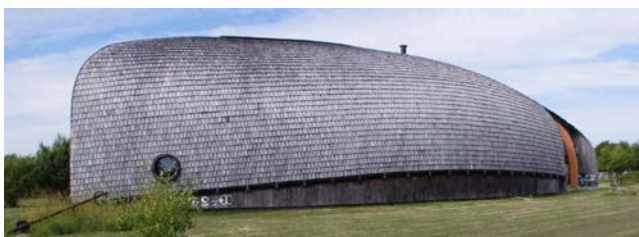
Triple-lapped chestnut roof shingles on the home and workshop of Jean-Noël Duchemin ('pêcheur de tons'), Beuzec-Cap-Sizun (France)
