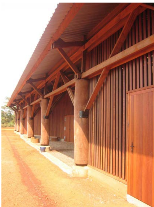
Door in Moabi, posts in Tali, framework in Kosipo, vertical thin timber cladding in Mukulungu – J.Y. Riaux, Mindourou (Cameroon).
