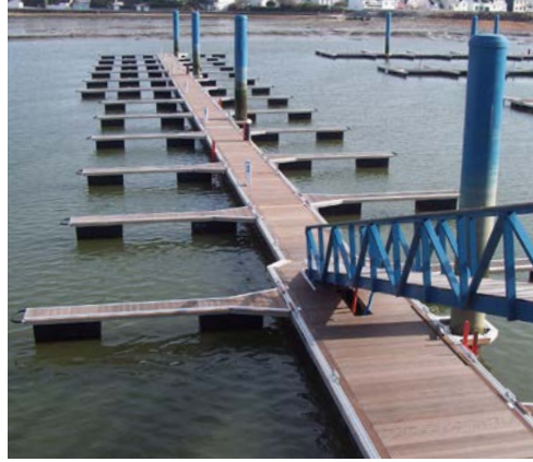
Floating decks, Port-Louis (France).
