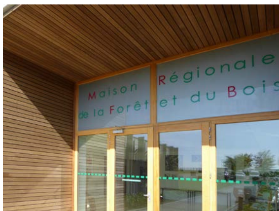
Outdoor covering (sheltered) in heat-treated Poplar, regional forestry and timber centre, Châlons-en-Champagne (France).
