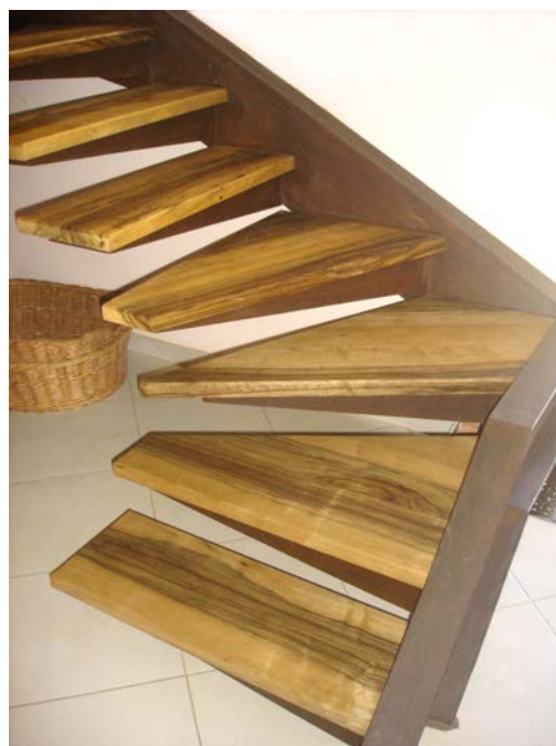
Semi-spiral, suspended staircase (in multi-coloured Fraké), Saint-Gély-du-Fesc (France).
